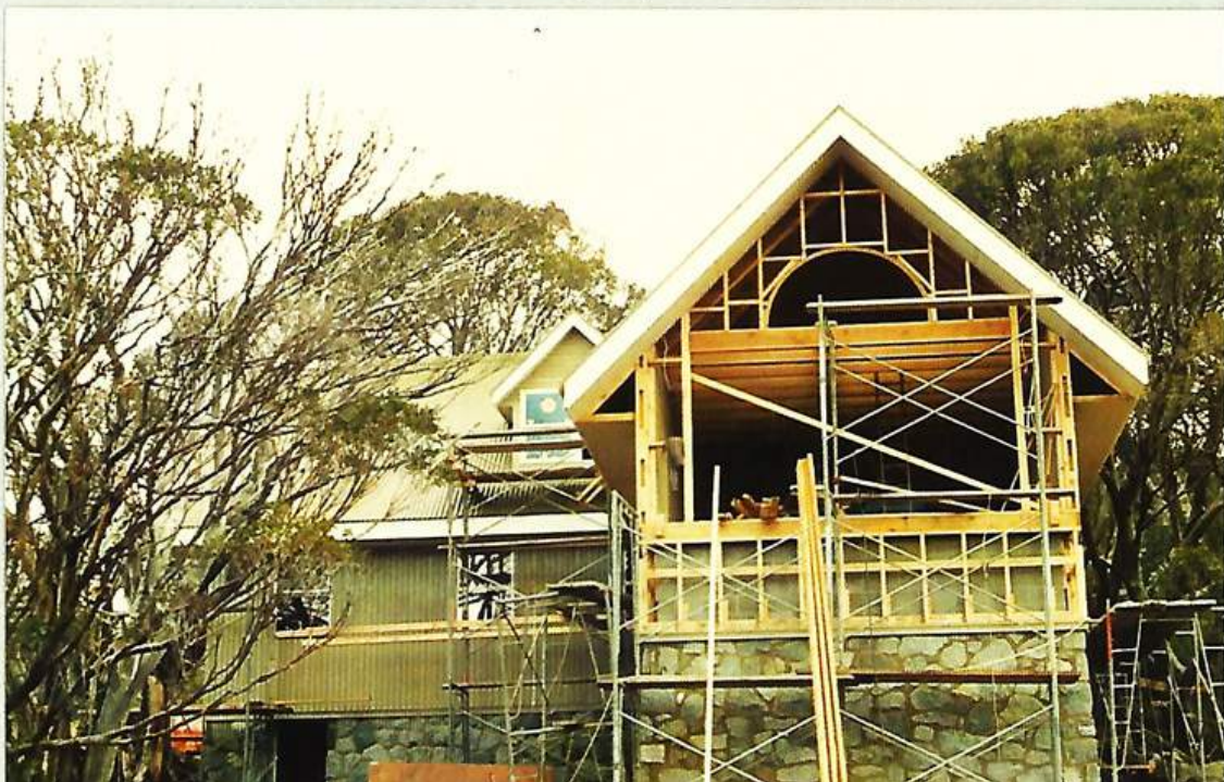
Extensive remodevation to DINELLA ski lodge completely gutted & refurbished, new roof & Extended out all new cladding replaced to outside
